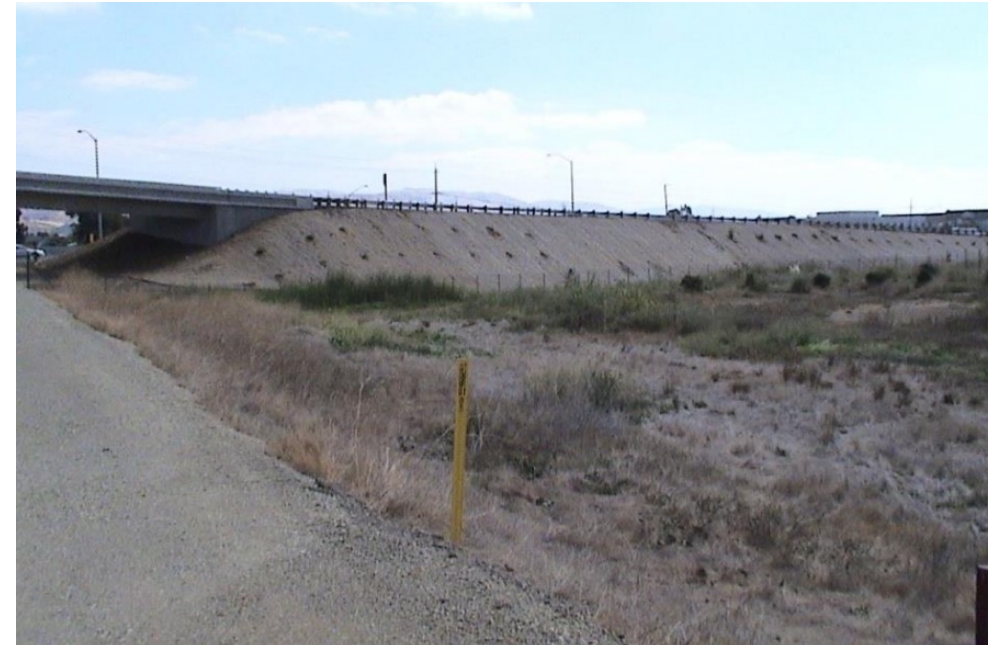
Final Dixon Landing TDA road embankment
