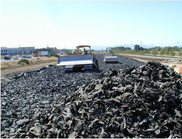
TDA being compacted at Dixon Landing, CA
