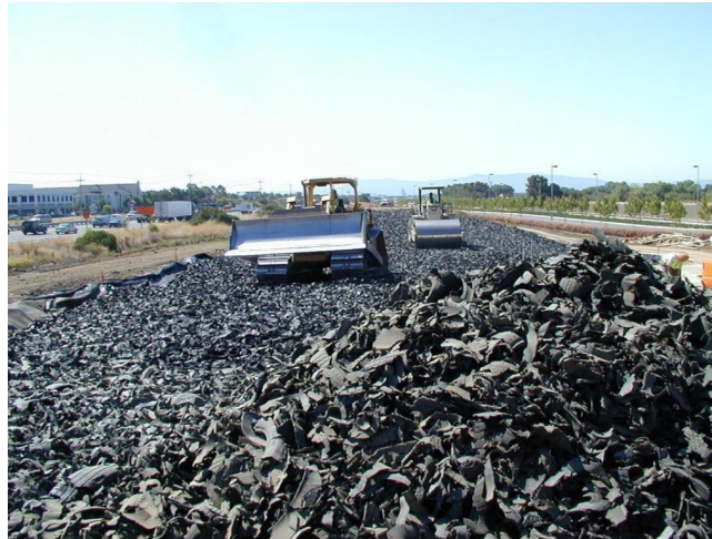
TDA- Road Embankment
