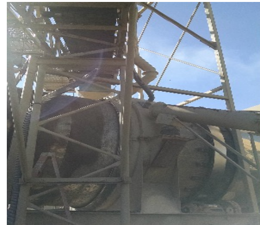
INJECTED THROUGH RAP COLLAR
