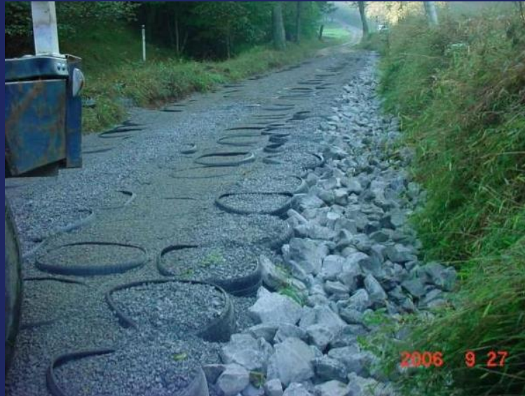
Rural road base course with 2" of wearing course surface aggregate
