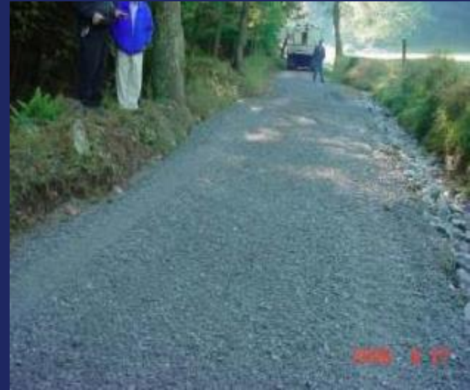
Rural road base course with 2" of wearing course surface aggregate
