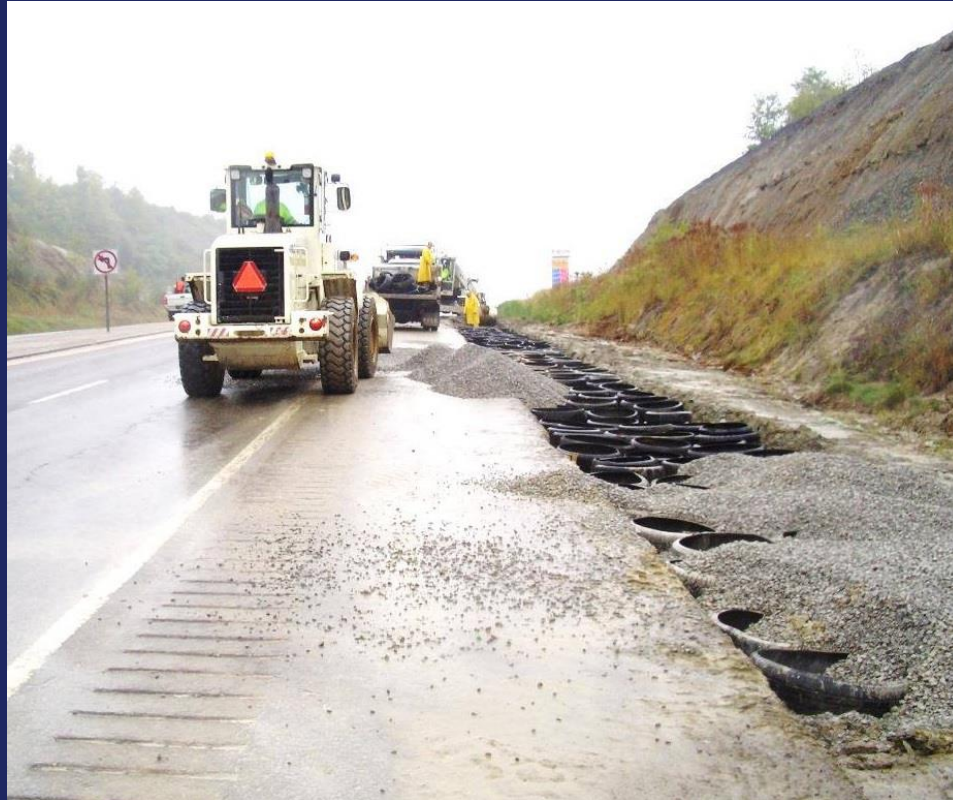
Highway shoulder stabilization & drainage solution
