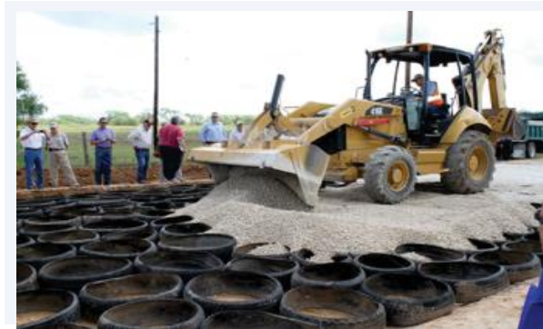
Cylinders Filled With Aggregate
