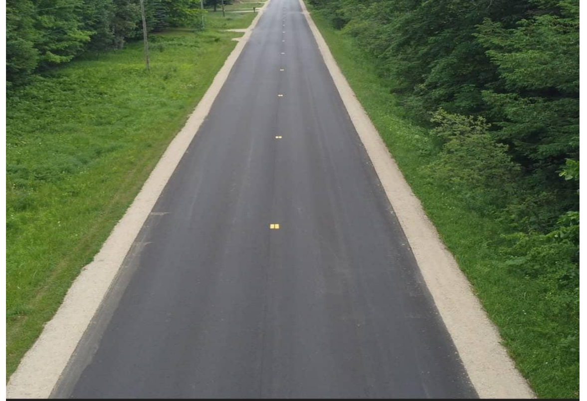
Reconstructed pavement surface (after construction)
