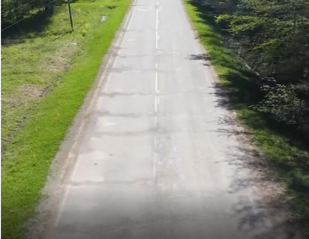
Original pavement surface (before reconstruction)
