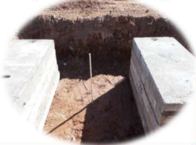
Setup1 (1.0m backfill with granular materials)
